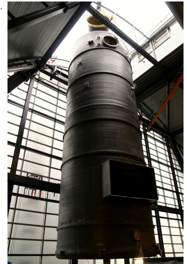
Scrubber during installation.
